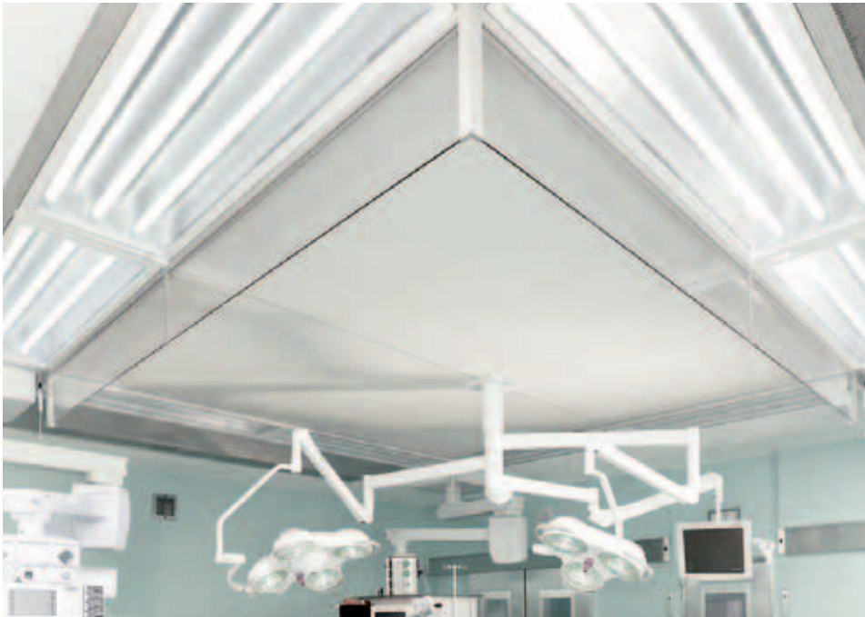
Weiss OT Clean Air Canopy. Photo courtesy of the pediatric cardiac center of the Justus Liebig University hospital, Gießen, Germany
