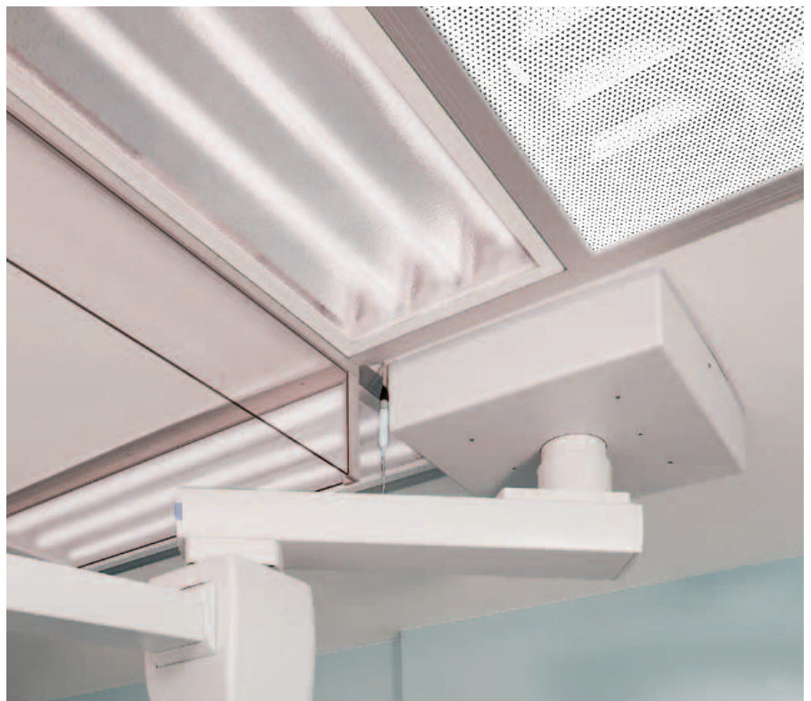
OT-clean air canopy with air-guide skirting of laminated safety glass or plexiglass. Hygienic recessed luminaires (protection class IP 65), circulating air suction of painted perforated sheet metal.
